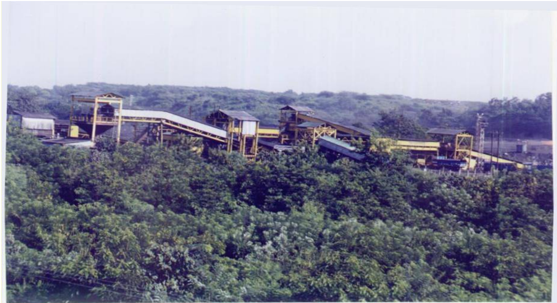
A BIRD'S EYE – VIEW OF CHP AT UMRER OCP
